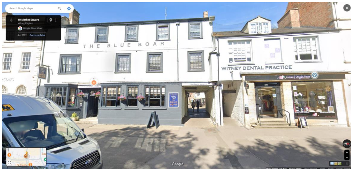
Looking west towards archway towards Marlborough Lane
